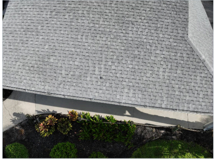
Photo 2: Front slope, eave and gutter line (nadir view)
