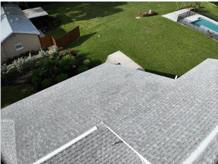
Photo 5: Oblique view of main roof field and valley over rear yard
