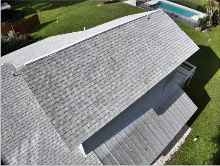
Photo 1: Rear slope overview with ridge vent and metal lean-to roof
