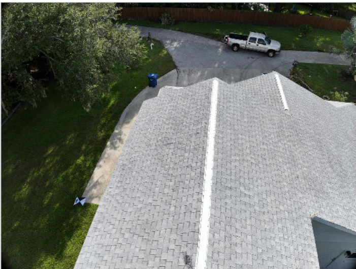
Photo 11: Front slopes and ridge vents over driveway
