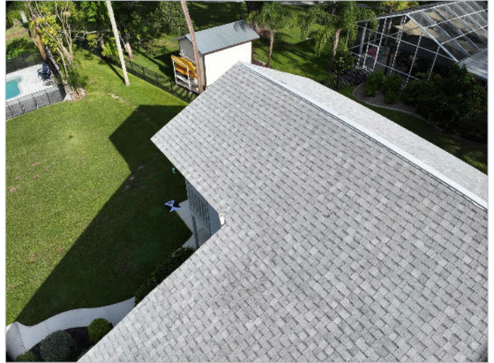
Photo 10: Side slope and valley, oblique view toward rear yard
